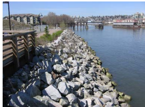
Dyke management in Queensborough to address Freshet water levels.
