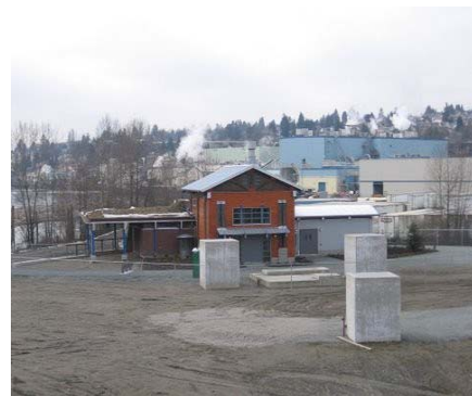
New Westminster's Combined Sewer Overflow (CSO) tank located within Muni Evers Park. Source: City Staff
