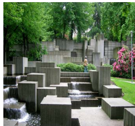
Park and open space created on a plinth as Freeway Park, Seattle, WA.
